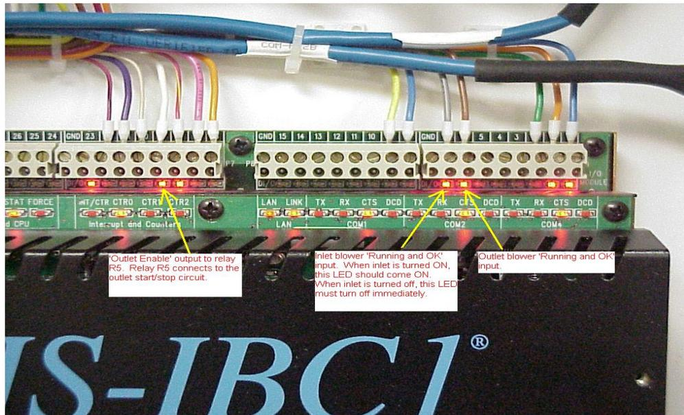
Figure 2 - Testing for Proper Operation of Inlet Blower Controls
